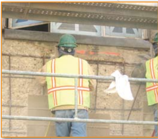
Figure 3: Jackhammer demolition in progress exposing corrosion damaged reinforcing bars.
