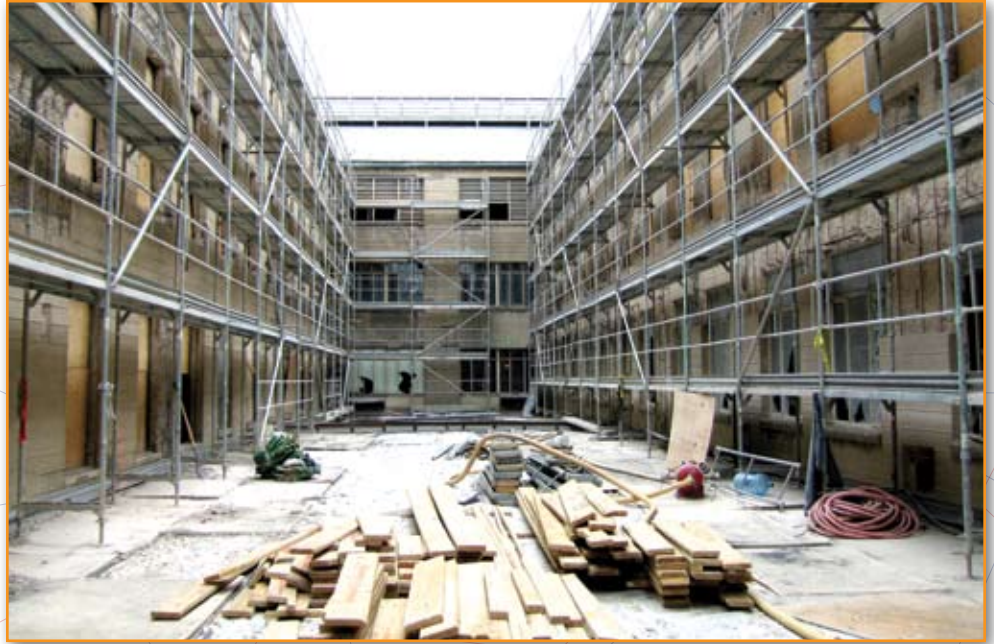
Figure 2: Scaffolding constructed to allow direct access to walls.
